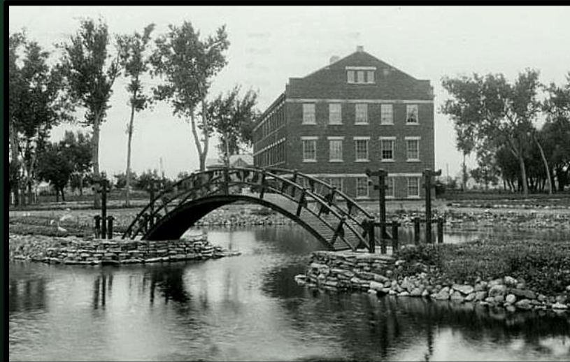
Pond bridge built - 1934
