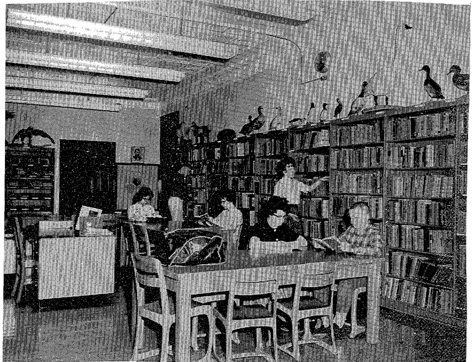
Library in the school building.
